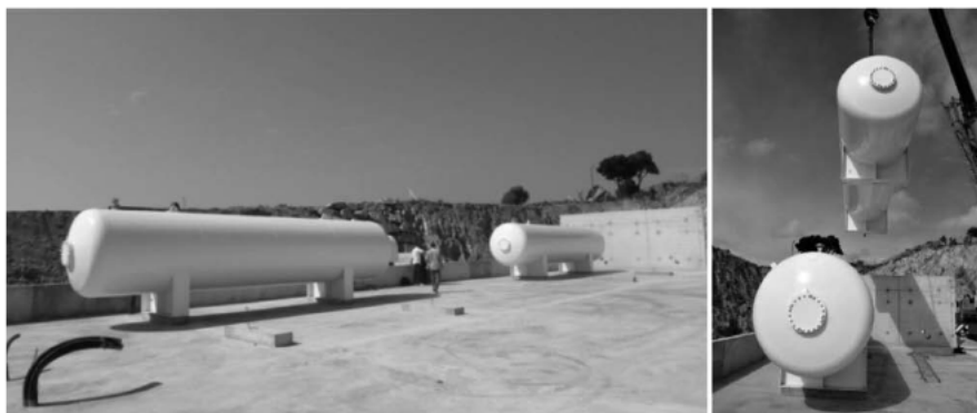
Figure 2.51. Installation of gas storage tanks on site [GAI 11]
