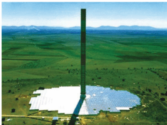
Figure 1.28 Solar - wind power station, 50 kW. (1982 - 1989, Manzanares, Spain).
