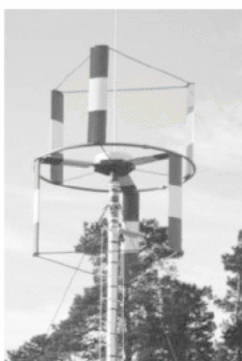
Figure 4.4 Modern balanced windmill (VAWT) 3 kW [3].
