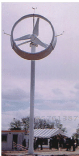
Figure 2.30 Wind unit with the diffuser concentrator, power 30 kW. France.
