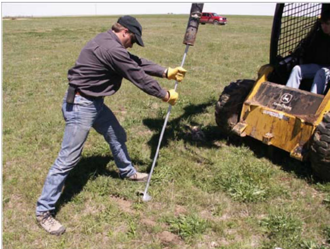
Figure 5-4. Example of a screw-in guy anchor installation. Source: AWS Truepower.
