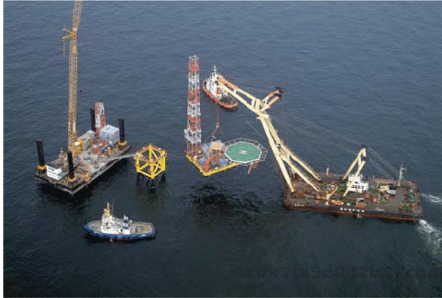
Figure 14-7. Installation of the FINO 1 offshore research platform using a jack-up barge (left) and a crane barge (right). Source: FINO 1 research platform, Copyright Bilfinger Berger Civil, Germany.
