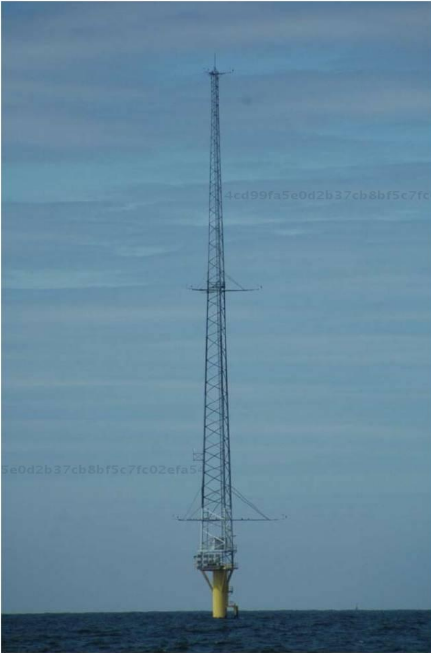
Figure 14-6. (a) Offshore meteorological tower for the NoordzeeWind project.
